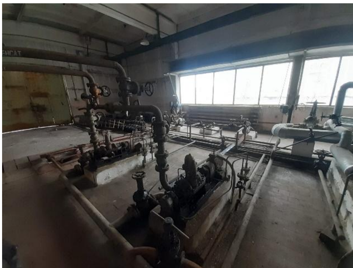
Figure 4.1.10. Condensate pumps
