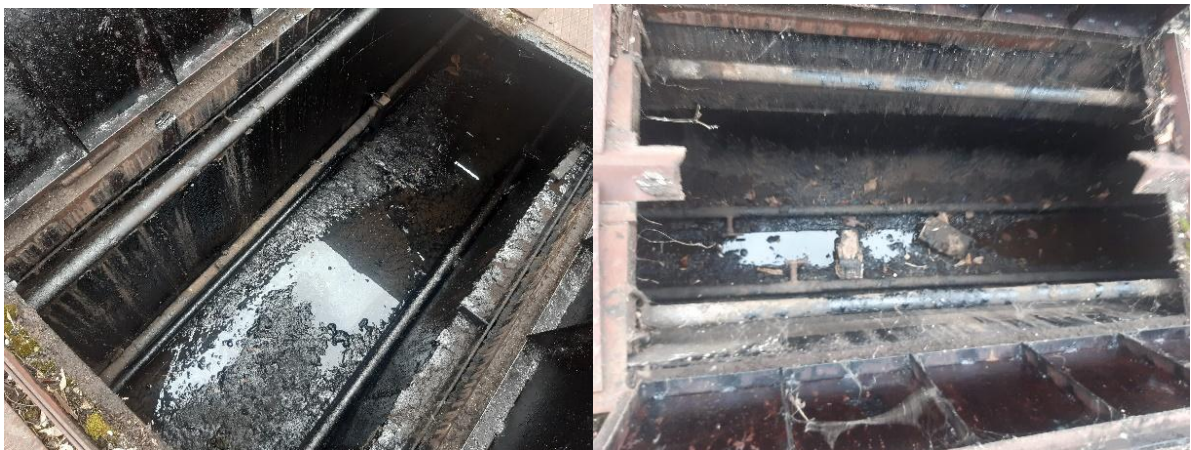
Figure 4.1.3. Mazut receiving and draining device/pits
