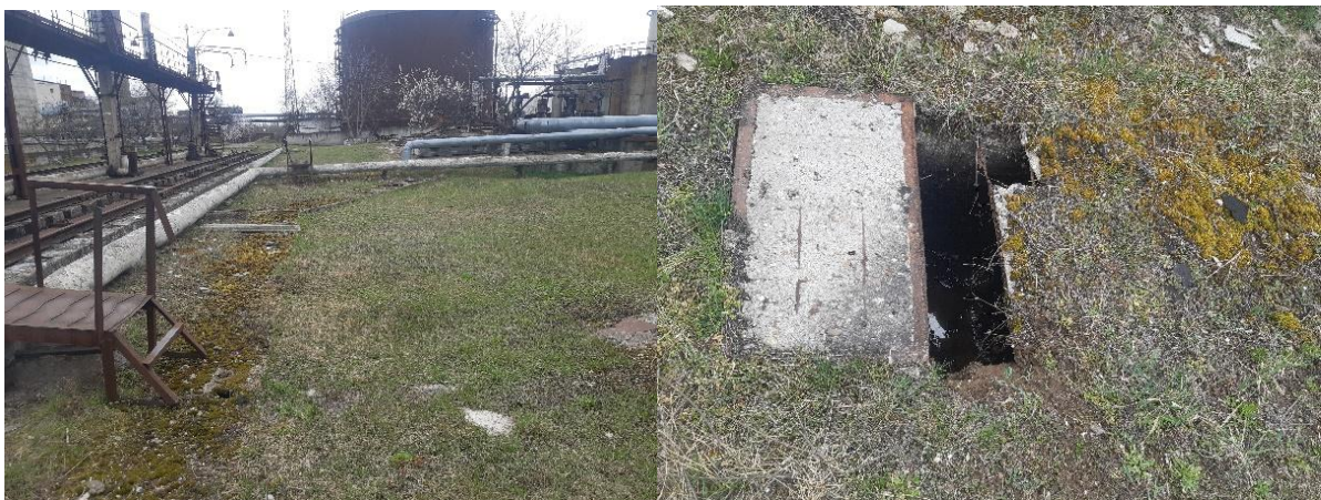
Figure 4.1.5. Concrete mazut drain channel
