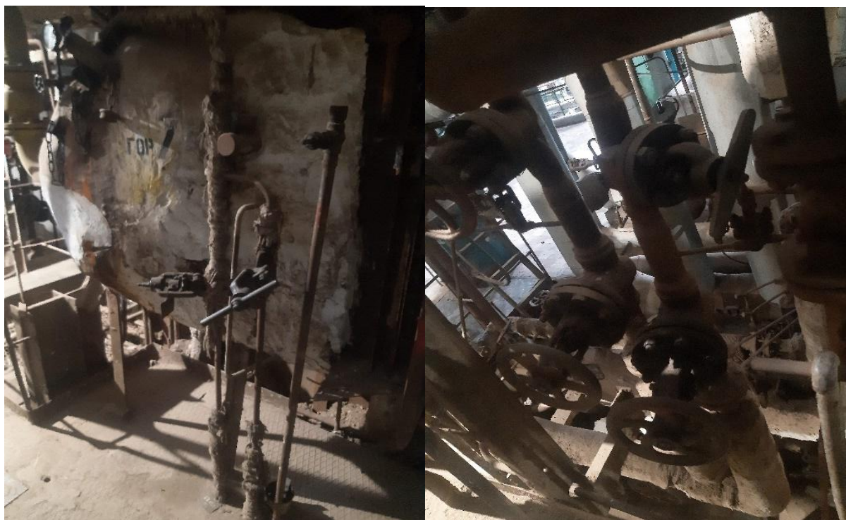
Figure 4.1.14. Mazut pipelines in boiler and turbine shop (boiler KA-4)
