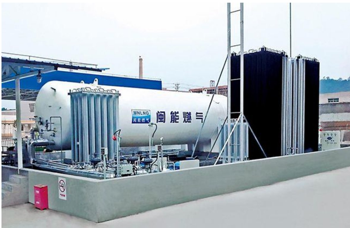
Figure 3.2.3. LNG cylinders produced by CIMC Enric (150 m 3 )
