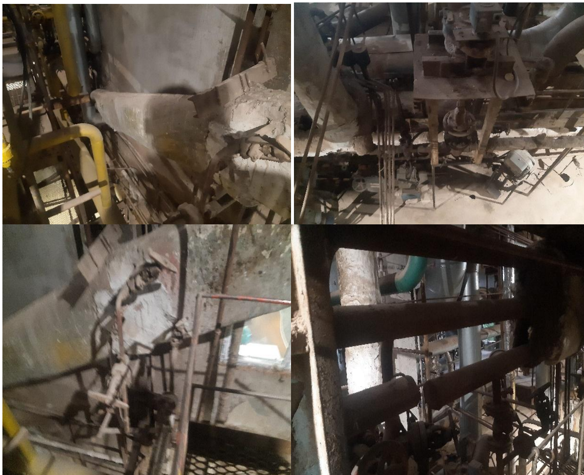
Figure 4.1.14. Mazut pipelines in boiler and turbine shop (boiler KA-4)
