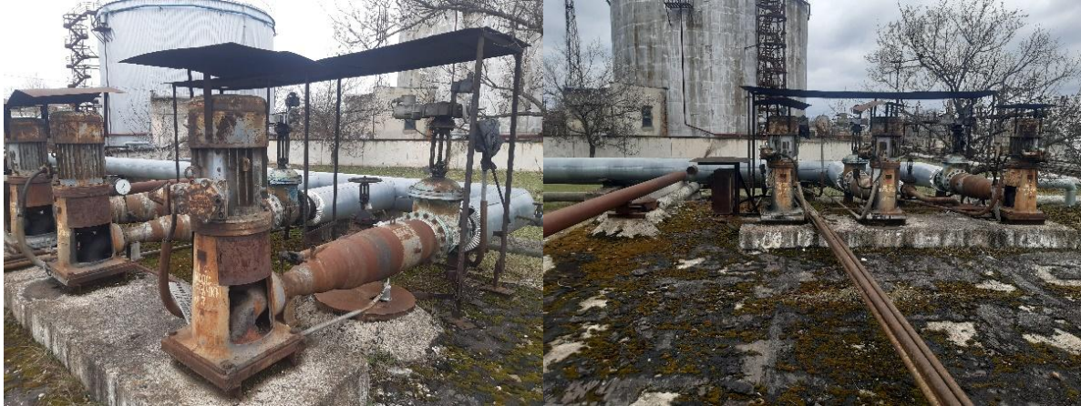
Figure 4.1.6. Transfer pumps МНП 1, 2, 3
