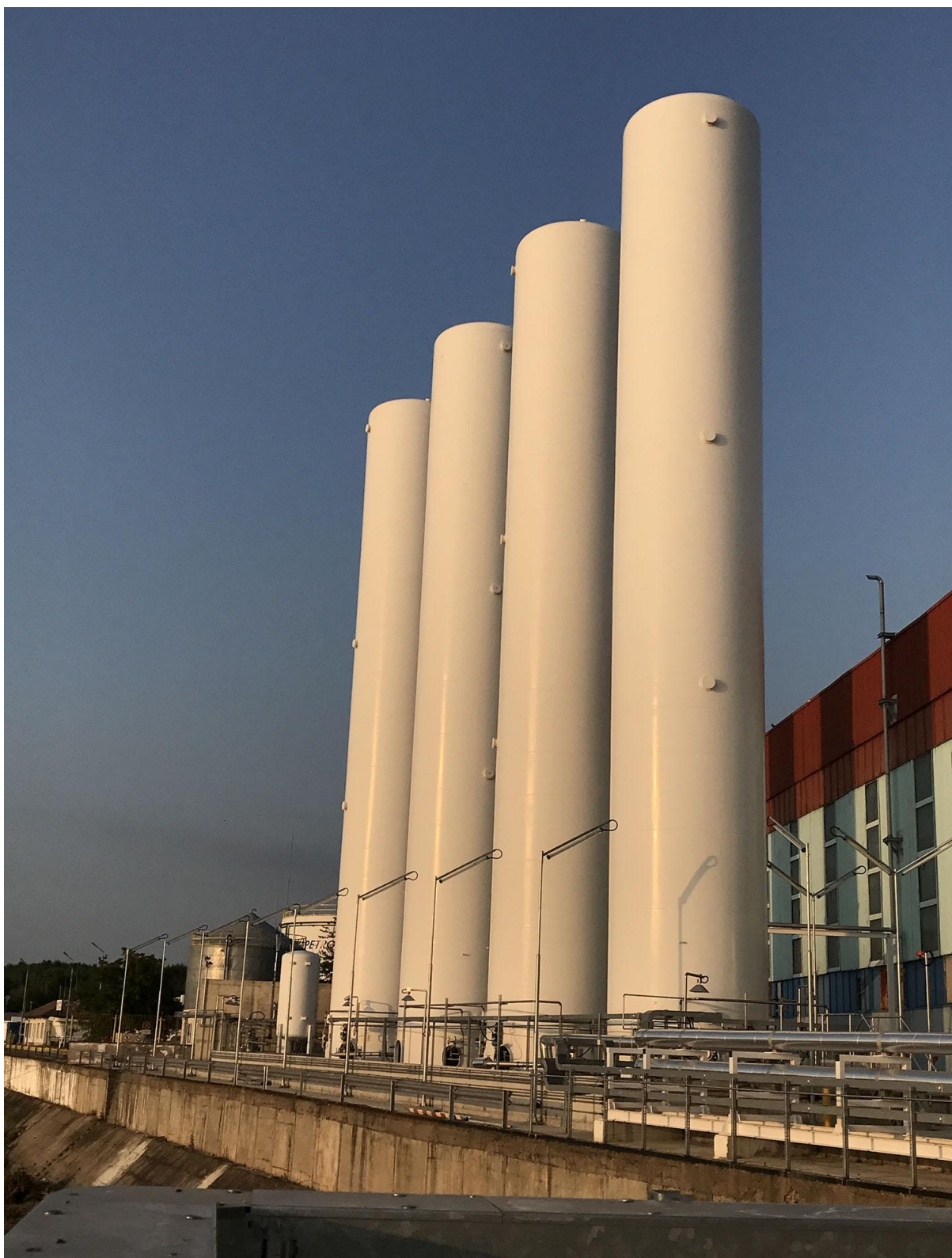
Figure 3.2.2. LNG cylinders built by Bulmarket Ruse, Bulgaria ( 250 \text{ m}^3 \times 4 = 1,000 \text{ m}^3 )
